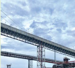
Controlling dust at bagasse storage facilities by spraying water and installing conveyor belt covers.
